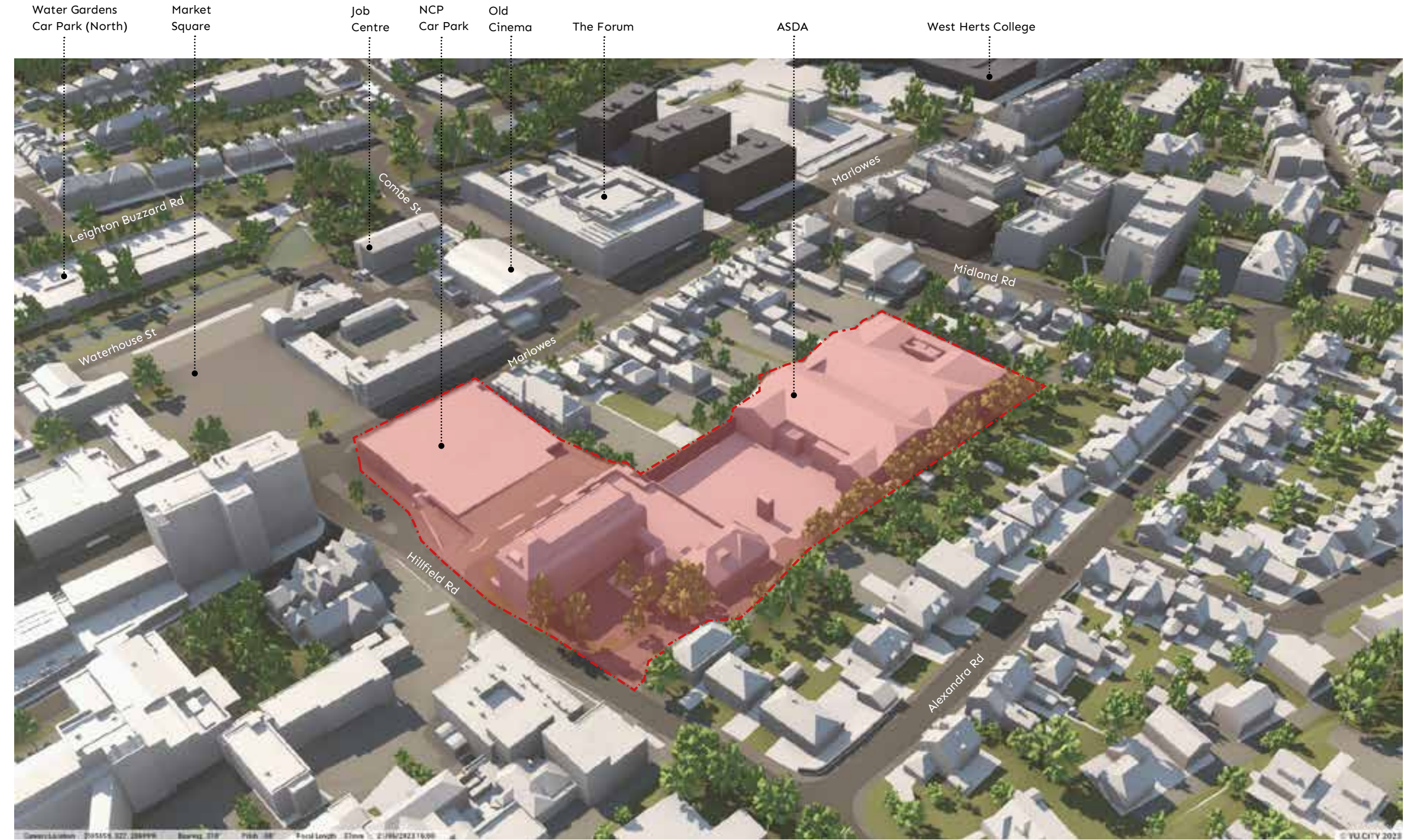
NCP car park, ASDA and Iceland site aerial view extracted from Hemel Hempstead 3D model produced by Vu.City
