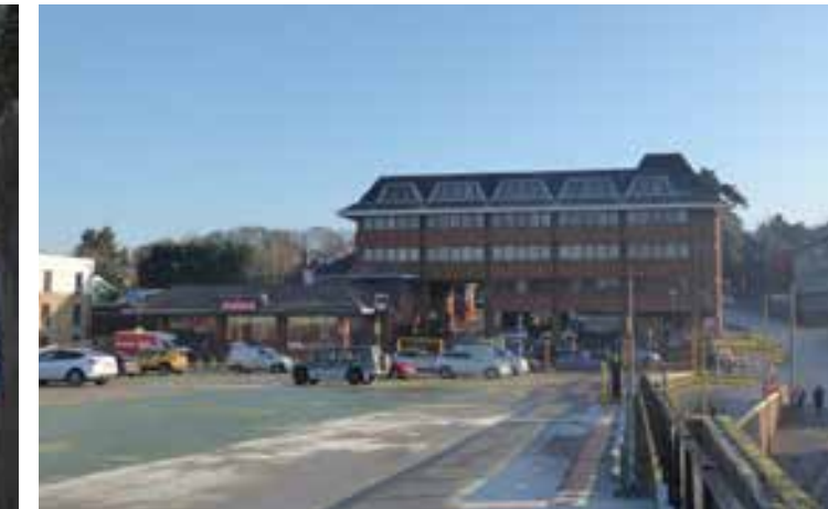
View of the office building from the NCP car park looking east
