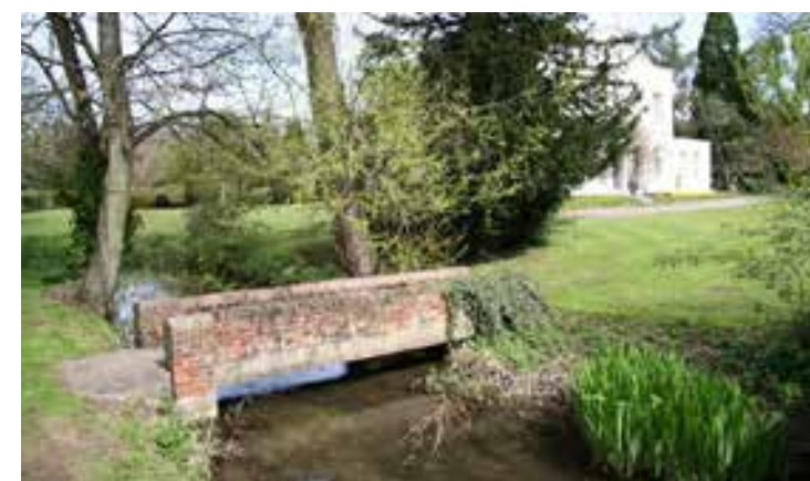
View of the Bury footbridge
