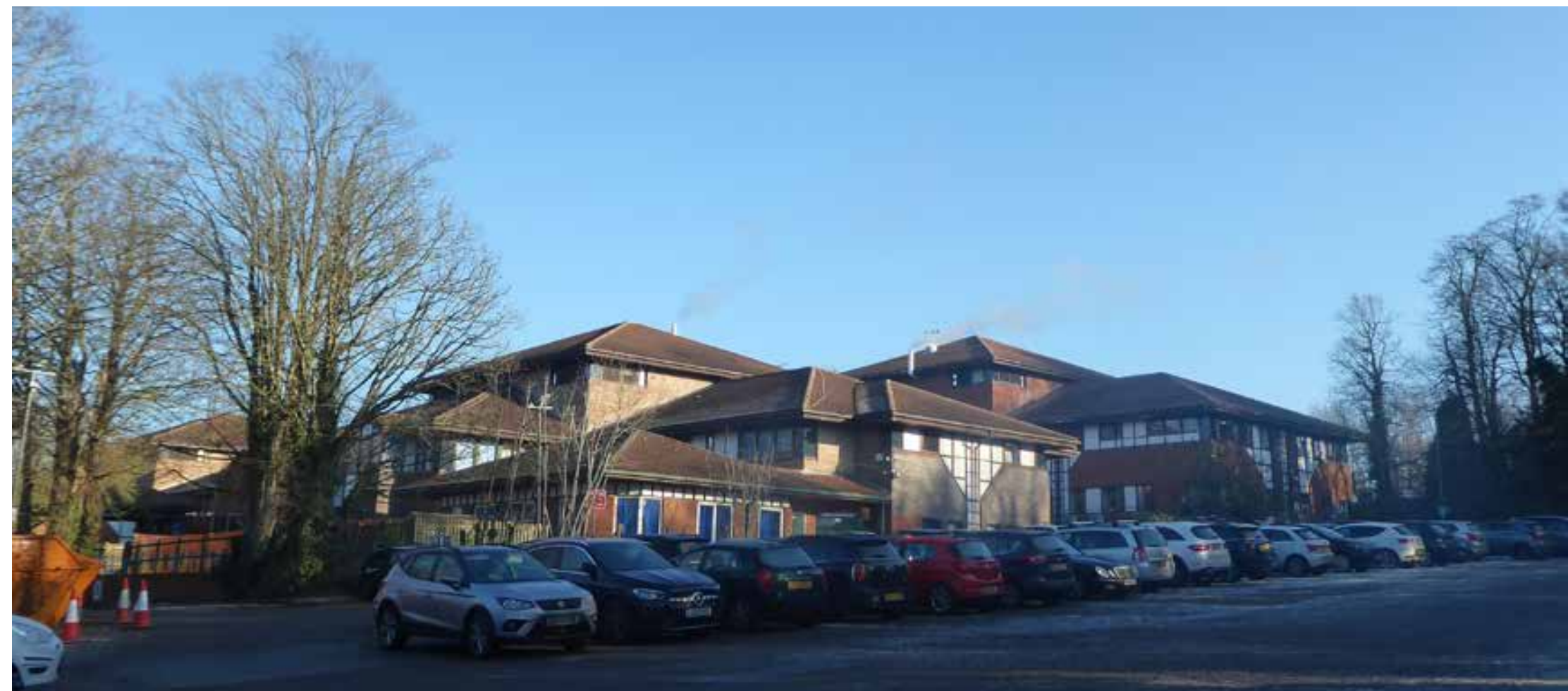
View of the hospital from the car park
